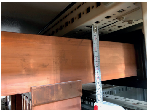
Support Profiles-Busbars
