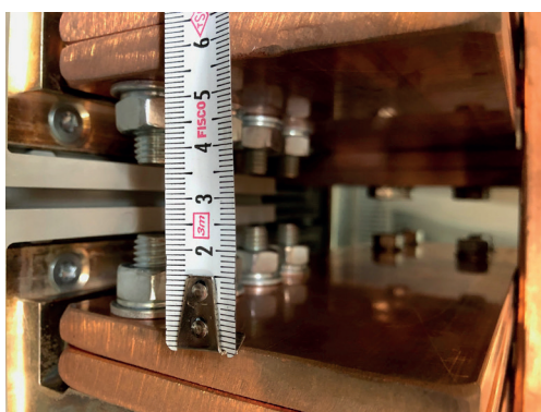
Breaker Connection Bolts
