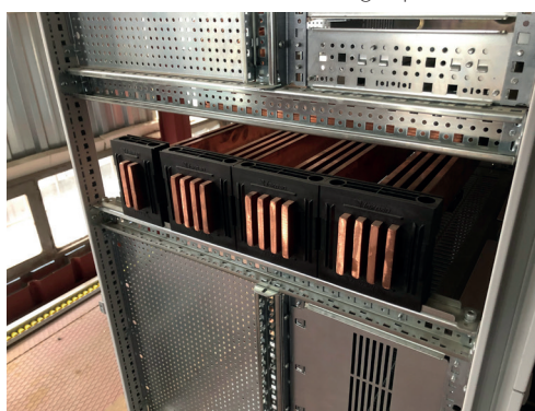
Busbars – Panel Joint Brackets
